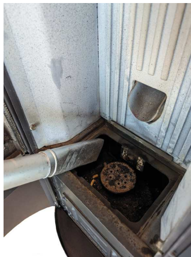
Fig. 55 - Vacuum out the ash
