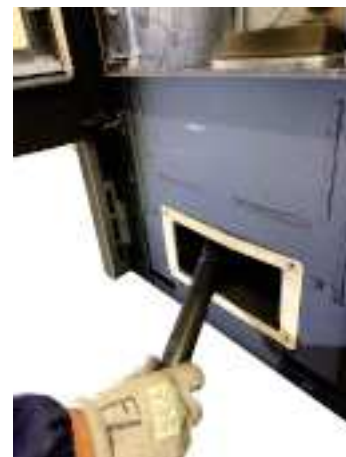
Fig. 67 - Vacuum out the ash
