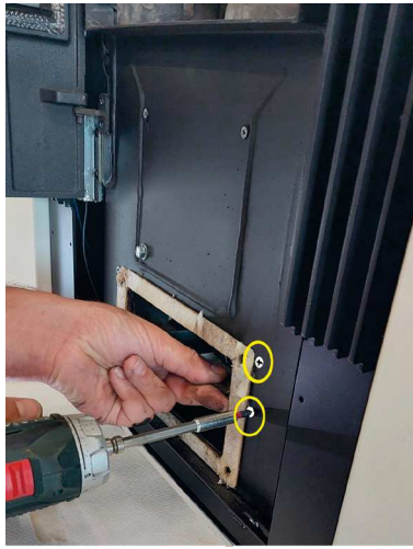
Fig. 69 - Unscrew the screws
