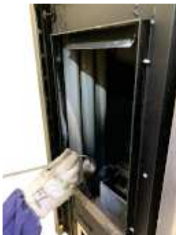
Fig. 66 - Clean with pipe cleaner
