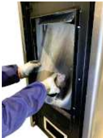
Fig. 64 - Remove the rear firebox panel
