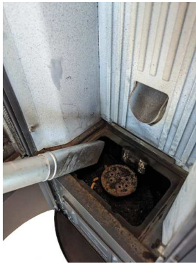
Fig. 74 - Burning pot box cleaning
