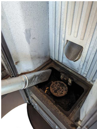
Fig. 31 - Burning pot box cleaning
