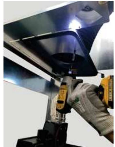
Fig. 69 - Flexible hose fixing
