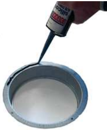
Fig. 68 - Silicone the flange
