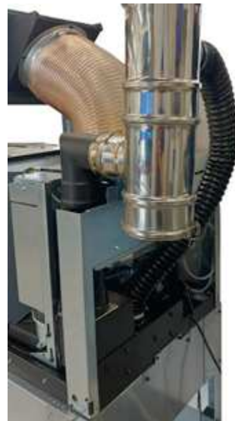
Fig. 80 - Concentric pipe connection + Combustion air
