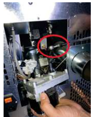
Fig. 89 - Gear motor removal
