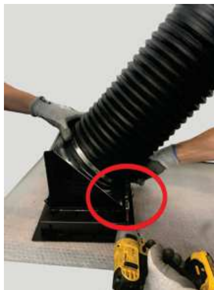
Fig. 65 - Tighten the clamp
