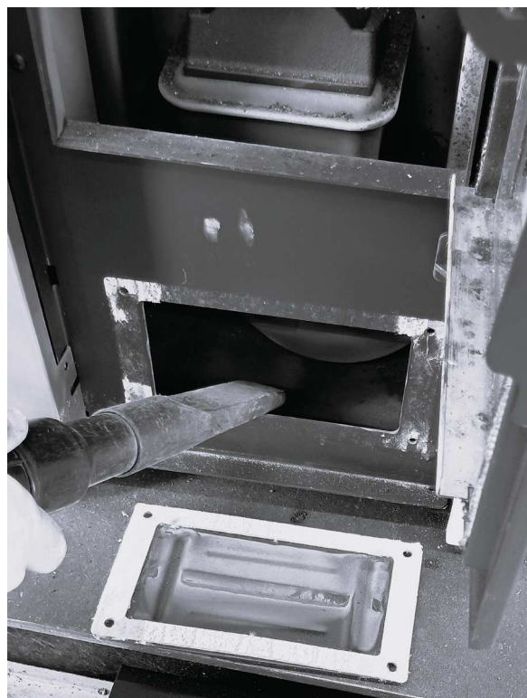
Fig. 29 - Vacuum out the ash
