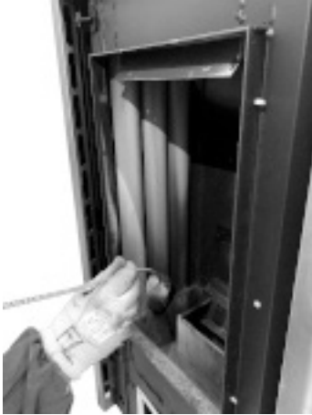
Fig. 60 - Clean with pipe cleaner
