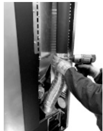
Fig. 38 - Fix the pipes
