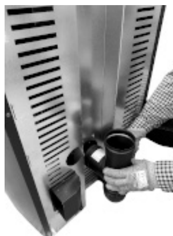
Fig. 22 - Connect the Tee fitting
