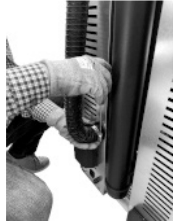
Fig. 28 - Insert combustion air pipe
