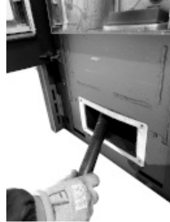
Fig. 61 - Vacuum out the ash
