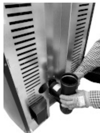
Fig. 22 - Connect the Tee fitting
