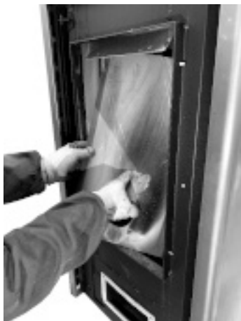
Fig. 58 - Remove the back panel of the firebox
