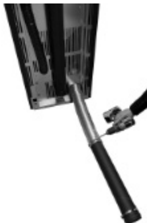
Fig. 38 - Connect pipe d.80 mm
