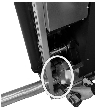
Fig. 37 - Block the flexible hose
