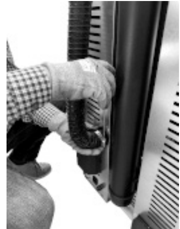
Fig. 28 - Insert combustion air pipe
