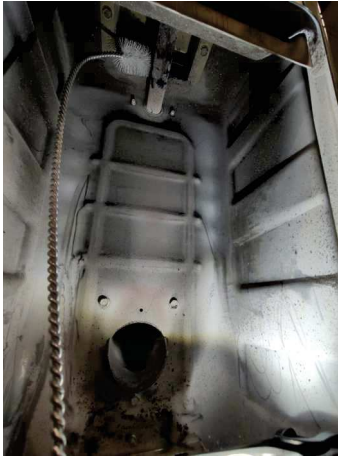
Fig. 81 - Clean with pipe cleaner
