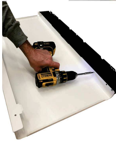
Fig. 41 - Fix the coloured side panel
