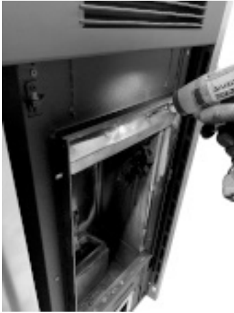
Fig. 117 - Remove the deflector
