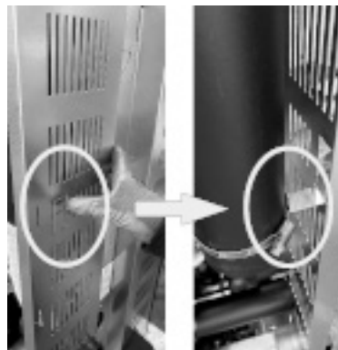
Fig. 84 - Fold the flap
