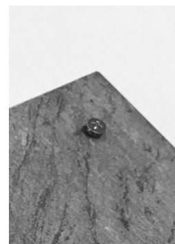
Fig. 59 - The screw must protrude
