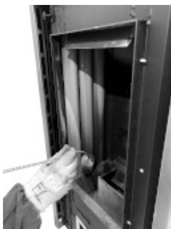
Fig. 123 - Clean with pipe cleaner
