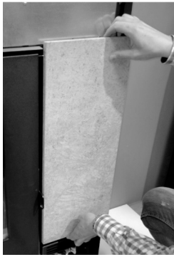
Fig. 60 - Hook the stone
