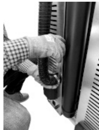
Fig. 75 - Insert combustion air pipe
