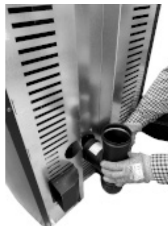
Fig. 69 - Connect the Tee fitting
