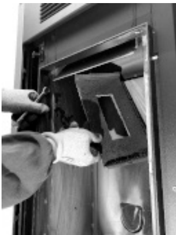
Fig. 120 - Remove the head of the firebox 2
