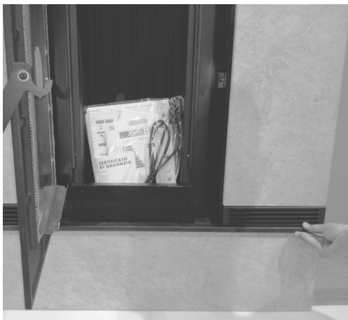
Fig. 63 - Position stone and profile
