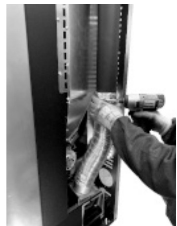
Fig. 85 - Fix the pipes
