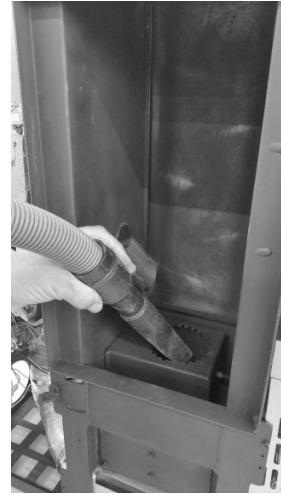
Fig. 59 - Vacuum out the ash
