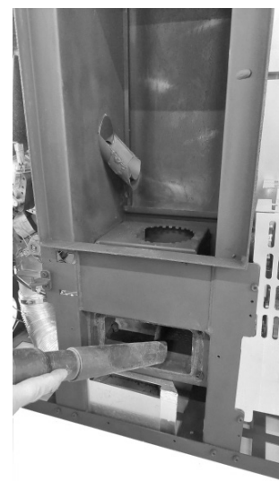
Fig. 64 - Vacuum out the ash
