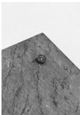
Fig. 22 - The screw must protrude
