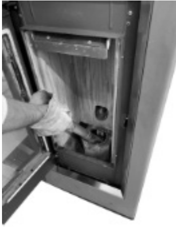
Fig. 33 - Burning pot box cleaning
