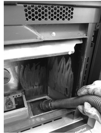
Fig. 27 - Vacuum out the ash
