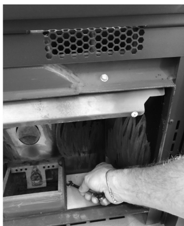
Fig. 24 - Remove the screws
