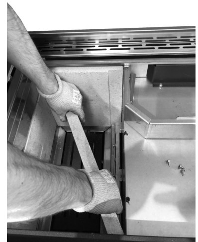
Fig. 68 - Remove the refractory material
