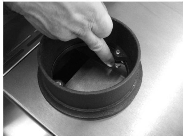
Fig. 46 - Fasten the stub pipe
