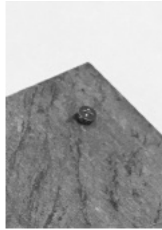
Fig. 29 - The screw must protrude
