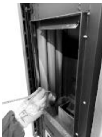
Fig. 124 - Clean with pipe cleaner
