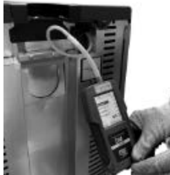
Fig. 109 - Digital pressure switch connection (Atena 3 Plus12/14 - Duke 12/14 At - Saba 12/14)
