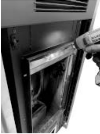
Fig. 118 - Remove the deflector
