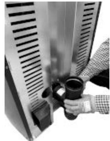
Fig. 70 - Connect the Tee fitting
