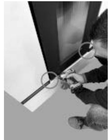
Fig. 47 - Fix lower panel
