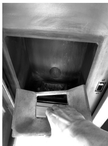
Fig. 59 - Vacuum out the ash
