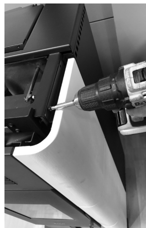
Fig. 29 - Securing the panel
