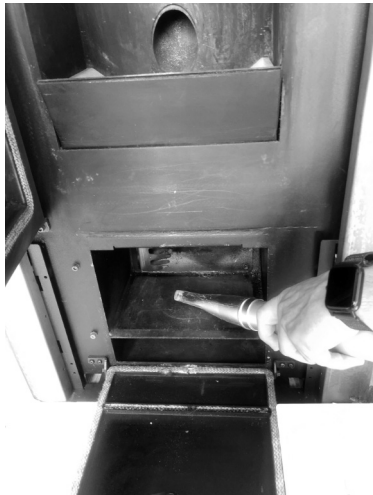
Fig. 61 - Vacuum out the ash
