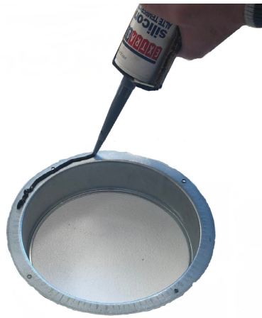
Fig. 68 - Silicone the flange
