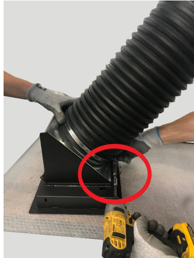
Fig. 65 - Tighten the clamp
