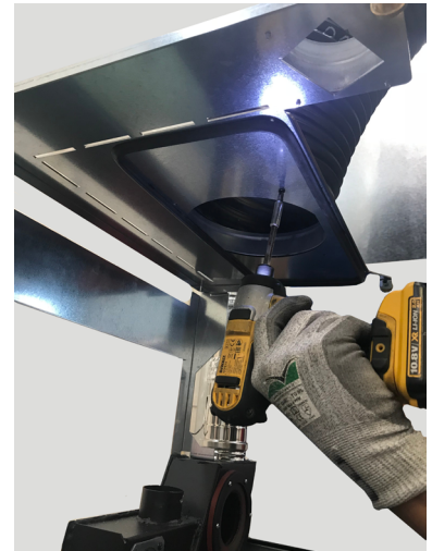
Fig. 69 - Flexible hose fixing
