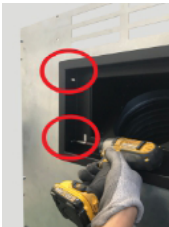
Fig. 70 - Trapdoor external fixing
