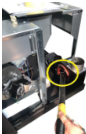
Fig. 115 - Smoke duct cleaning
