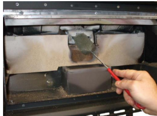
Fig. 49 - Clening with a brush
