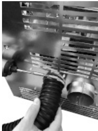
Fig. 12 - Raccordement air comburant
