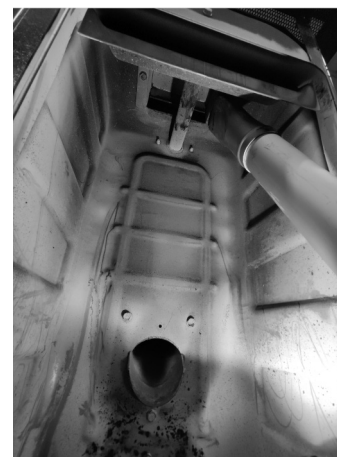
Fig. 73 - Vacuum out the ash
