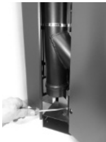
Fig. 66 - Unscrew the Cap stopper
