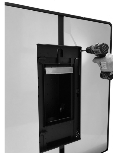
Fig. 38 - Coating fixing
