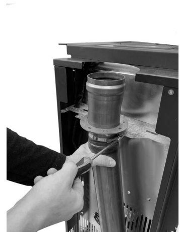
Fig. 42 - Block with clamp
