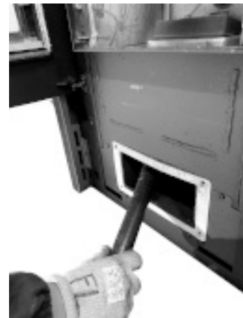
Fig. 82 - Vacuum out the ash
