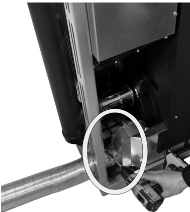
Fig. 66 - Block the flexible hose
