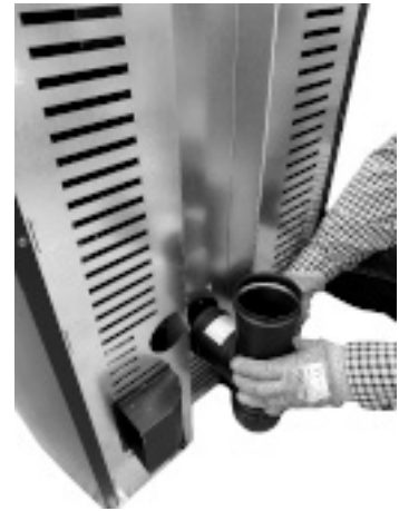
Fig. 51 - Connect the Tee fitting
