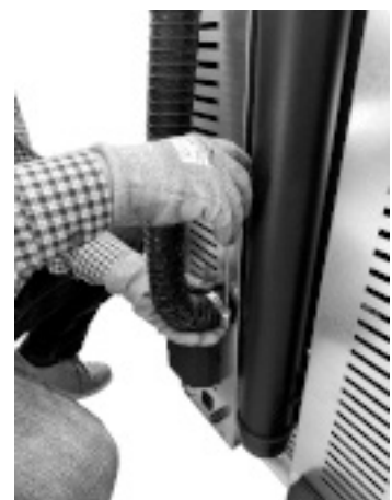
Fig. 57 - Insert combustion air pipe
