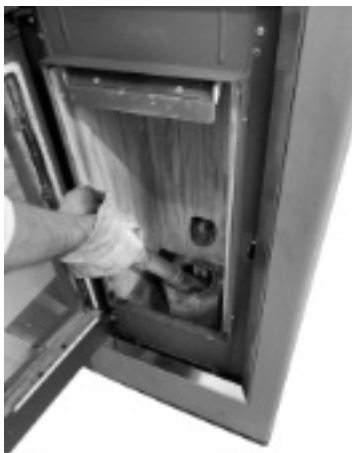
Fig. 35 - Burning pot box cleaning
