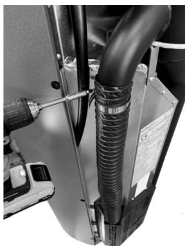
Fig. 78 - Remove flexible hose
